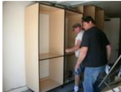
Carl & Jody installing cabinets in the Collman Communication Center
