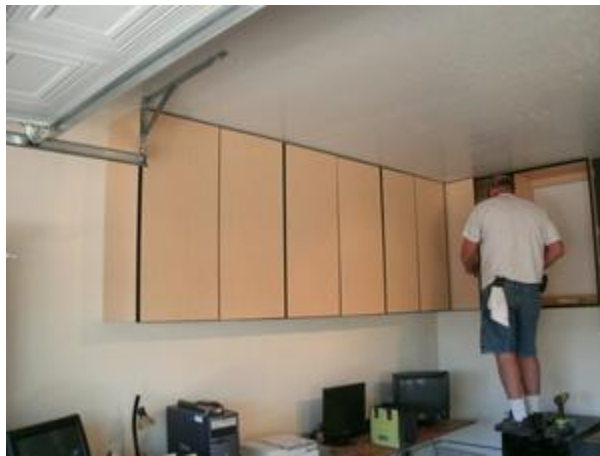
Carl installing cabinets in the Home Depot Lounge
