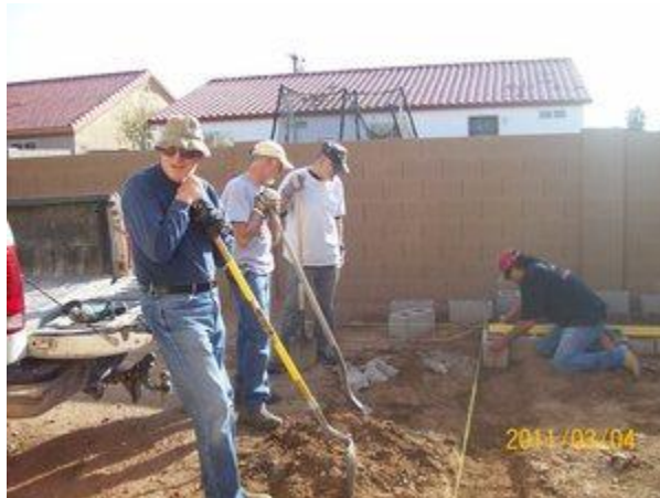
Building the foundation for the Shed
